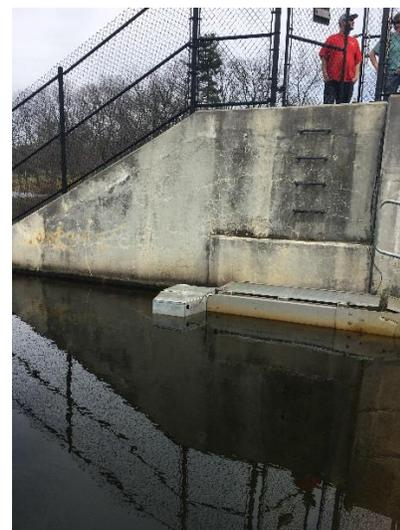
*The exit of the Bunnells Pond Fishway on the Pequonnock River in Bridgeport. This is the top end of what may be the tallest steepass fishway in the region. The spillway is to the right. The lighter silver box at the end of the fishway is the housing for our video camera. Images are analyzed by our partners at the Beardsley Zoo and streamed on-line. We'll share that link with you in a future report.*
